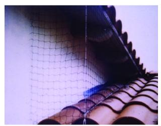
StealthNet used to exculde birds from the roof of a home
